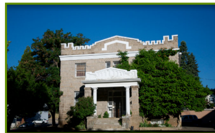
Figure 3-2 Old Lassen County Jail
