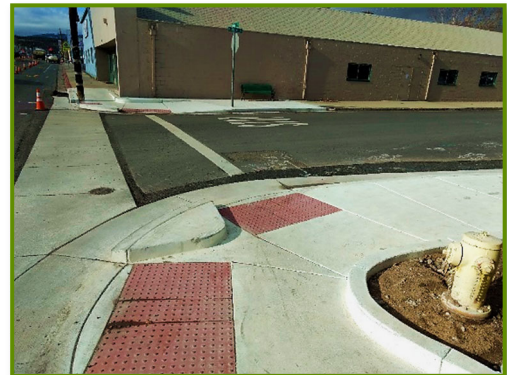
Figure 5-5 Caltrans CAPM Installed ADA Ramps
